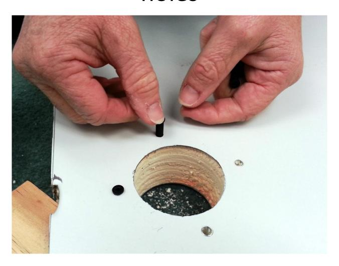
Place the Pipetite over the pipe penetrating the panel. (The plastic inserts are already placed into the holes)
